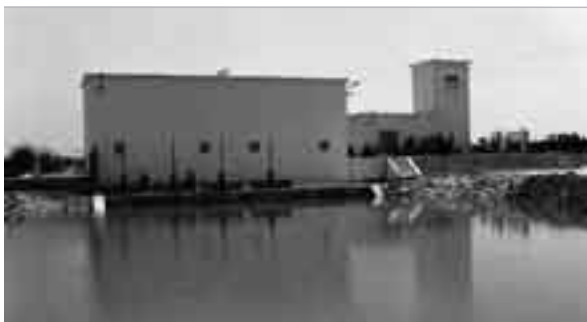
All drainage effluent from the Boudoum catchment area empties into the Gaëla drainage station (on the photo), from where it is discharged into the drainage channel of the Senegal river delta. (Photo: Madine Ndao, CIC/SAED)
